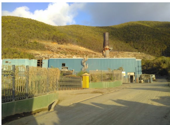
Photo 3: View of the incinerator
