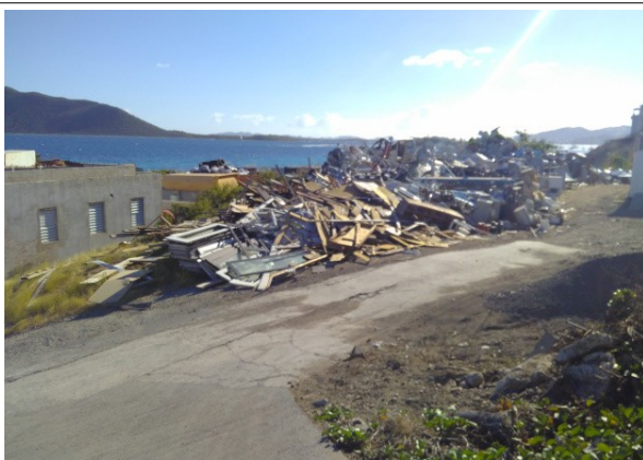
Photo 1: Hurricane debris on Scrub Island
